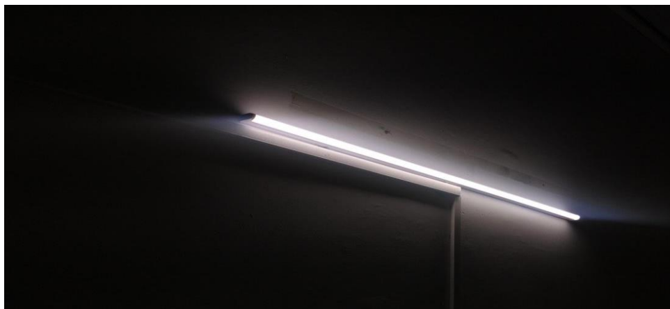
Photo: Replacement of Conventional Tube lights with LED Tube
