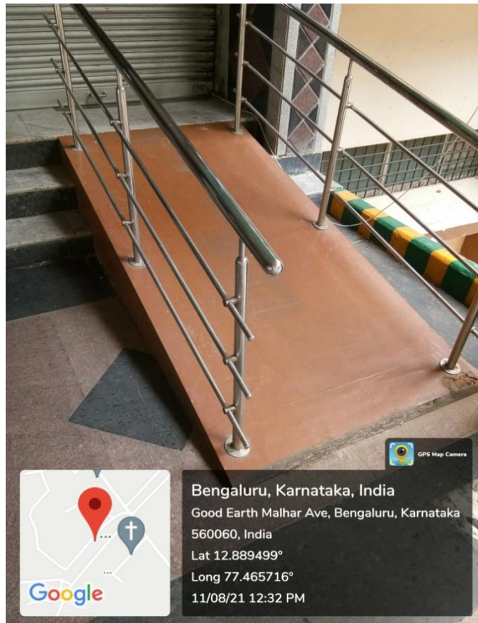
Photo: Ramp with Rails
