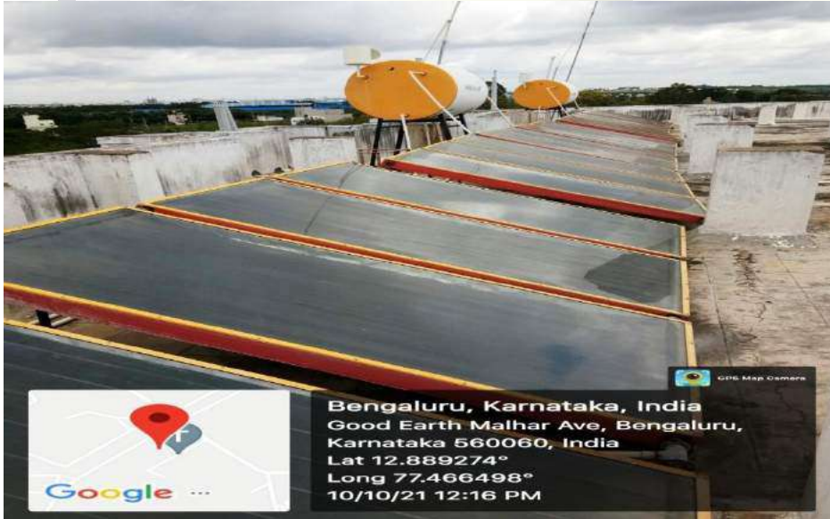
Photo: Solar Panels for water heating
