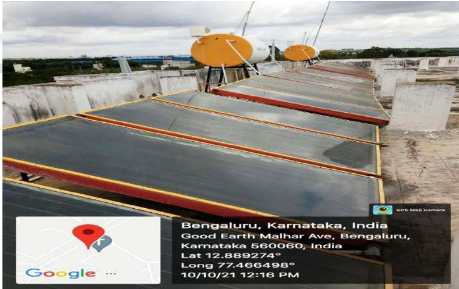
Photo: Solar Panels for water heating
