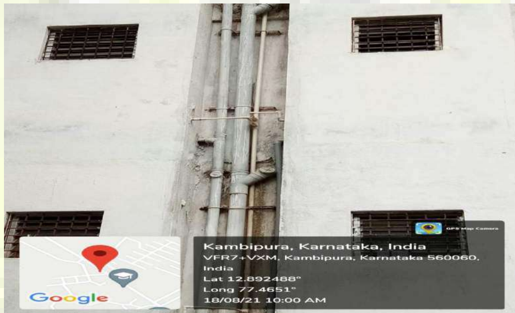
Photo: Water Bodies Distribution Line in the campus building
